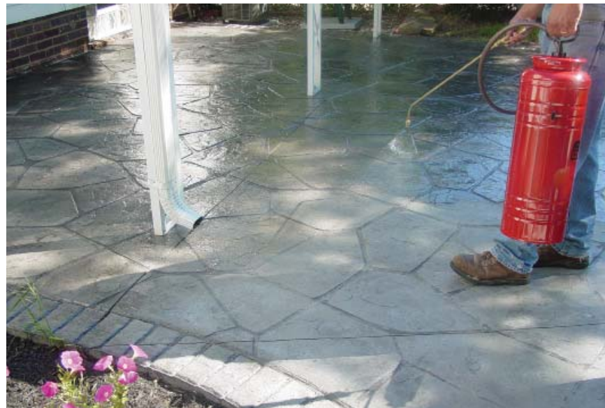
Common film forming sealers like cure & seals are applied in thin layers and typically last one to two years. Penetrating sealers can last as much as 10 years before reapplication is required.
