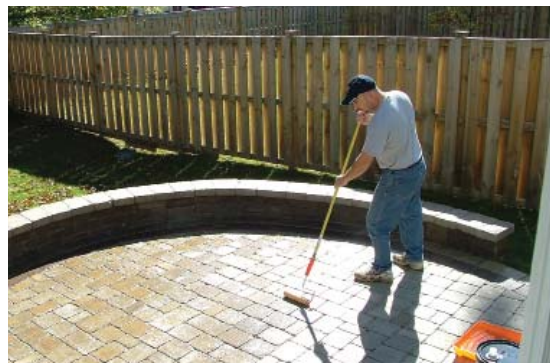
Water-based sealers, unlike solvent-based sealers, are sensitive to moisture and humidity during application and while in service.
