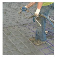
The American Concrete Institute specification 548.13-14 Bonding Fresh Concrete to Hardened Concrete with a Multi-Component Epoxy Adhesive requires that materials comply with ASTM C 881, Standard Specification for Epoxy-Resin-Base Bonding Systems for Concrete. However, the scope of ASTM C 881 only includes two-part epoxies, thus C 881 is not applicable to three-part epoxy/cement bonding systems. In spite of that, ASTM C 881 is still a good measure of performance for epoxy bonding materials.
